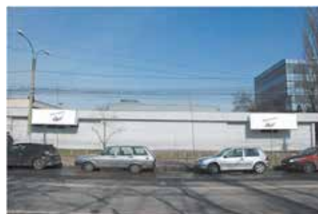
BANNER DISPLAY ON ROMEXPO HEADQUARTER FACADE
